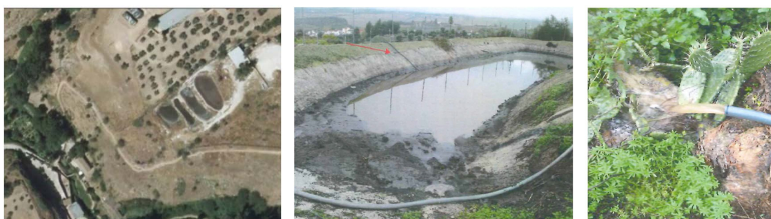
Figure 7.3.2.1. Photographs of the slurry ponds in Arriate and detail of an illegal emptying hose
